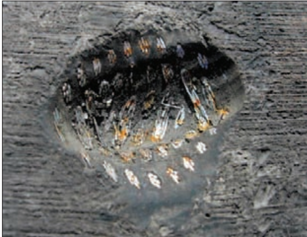
EFFECT: Exposed Steel Cord CAUSE: Detachment of Repair Product
