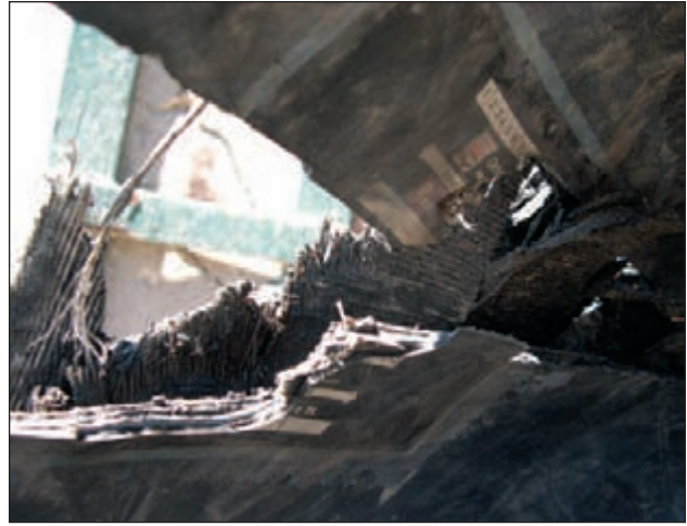
Rupture on Improperly Aligned Repair (Note that the arrows on the patch do not point toward the beads.)
