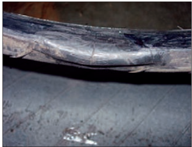
Bad Bead Repair
